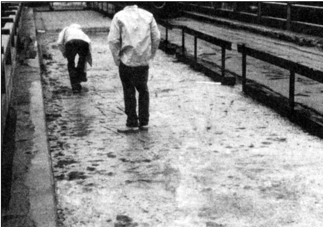
Exhibit X. 6 Surface Removed for Overlay
