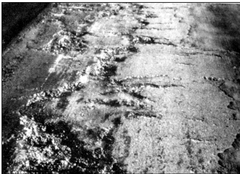
Exhibit X. 1 Deteriorated Deck
